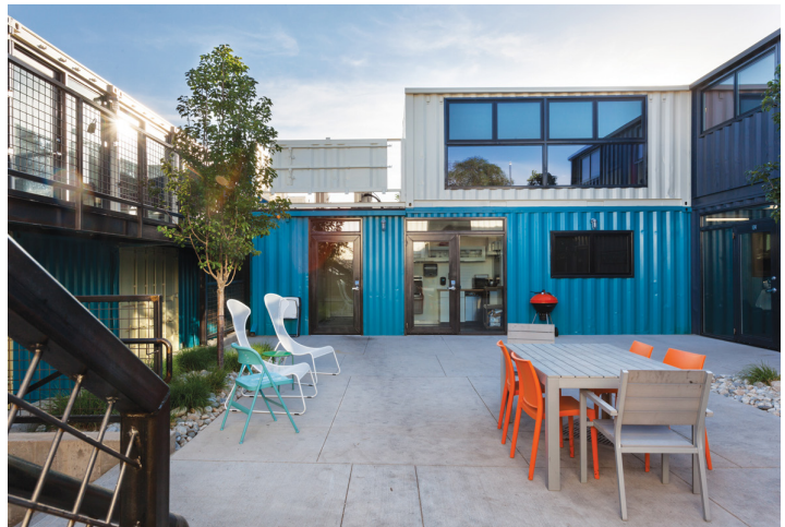
Made from custom-assembled shipping containers, the Gravitas development at 25th and Larimer in Denver is an example of “industrial modern” retail/office architecture.
